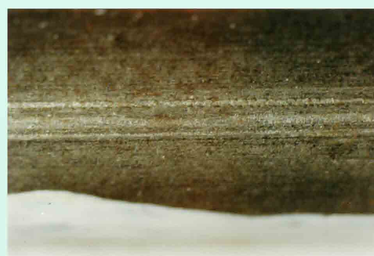
Surface after mechanical descaling with guidance marks
